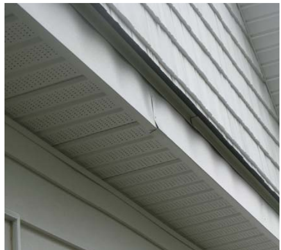
Aluminum coil wrap can dent and become wavy due to temperature changes.
